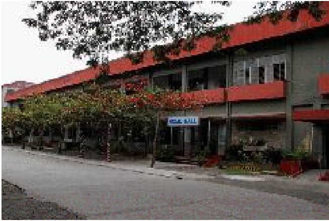
REPAINTING OF ROOFING (QUEZON HALL & EDUCATION BUILDING)
